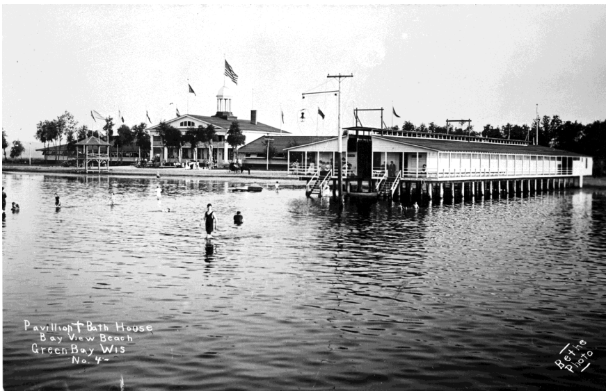
Bay Beach Pavilion and Bath House Photo #2648
